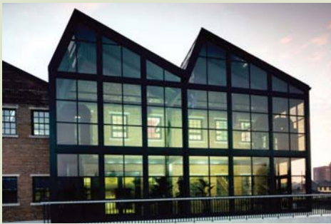
Bloomington City Hall and Showers Building
